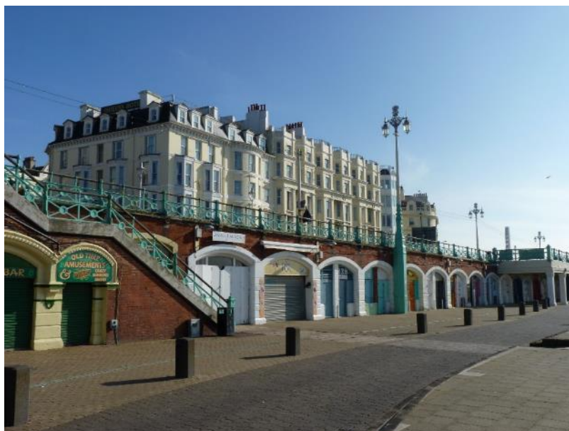
Brick arches supporting King's Road
