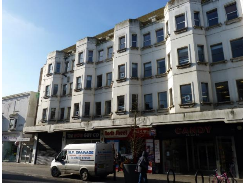
Nos.21-25 North Street
